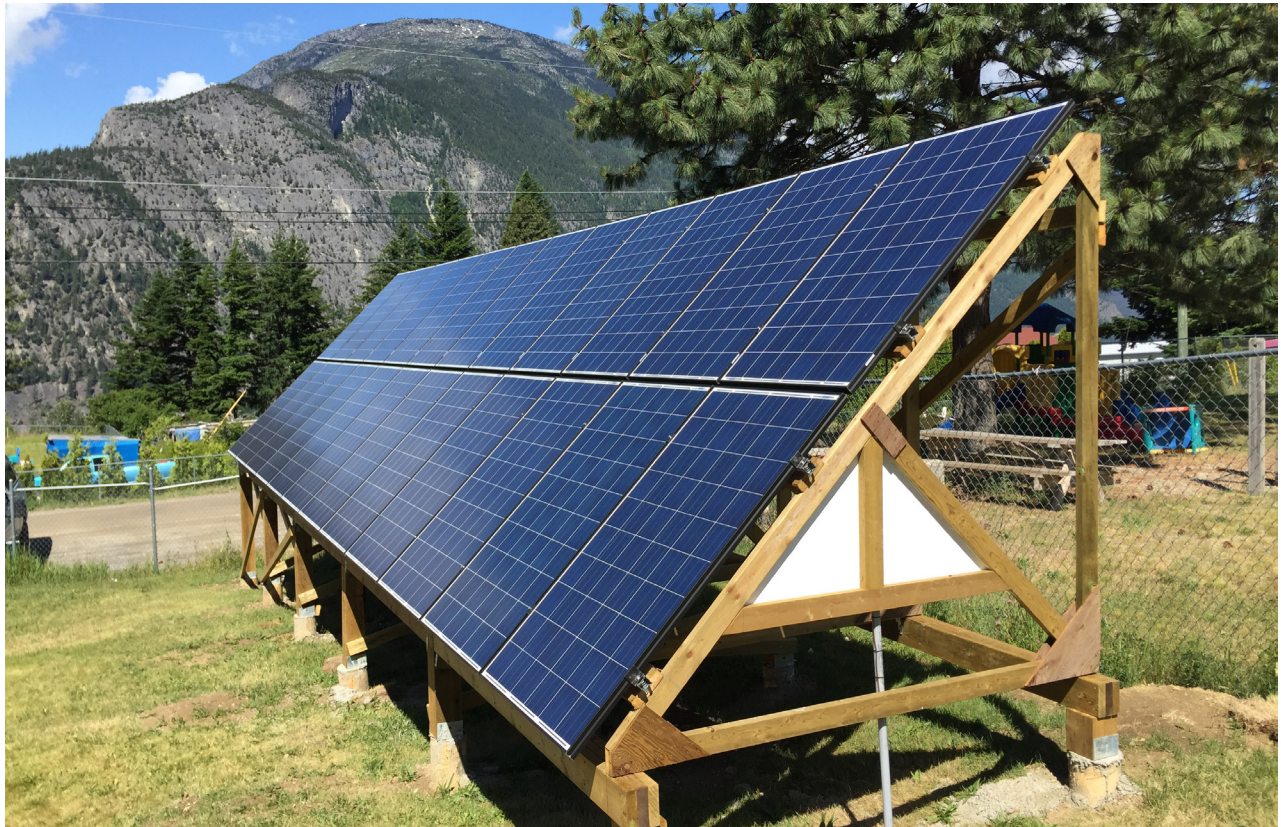
Ground-Mounted Solar PV System
