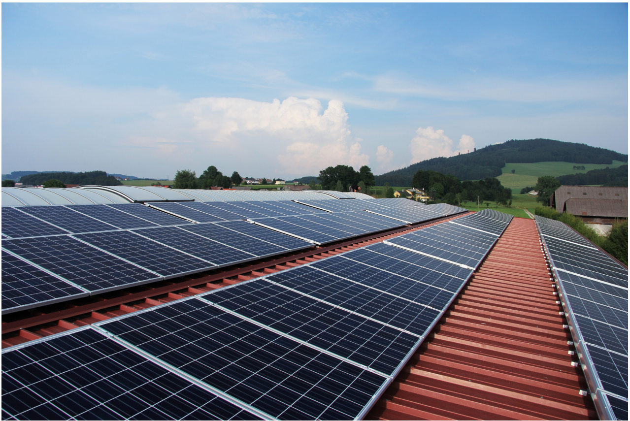
Roof-Mounted Solar PV System
