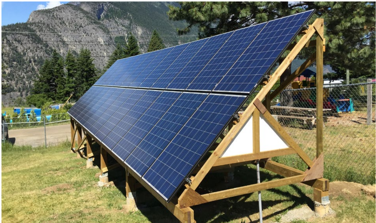
Figure 6-3: Ground-Mounted Solar PV System
